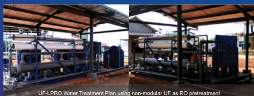
UF-LPRO Water Treatment Plant using non-modular UF as RO pretreatment
